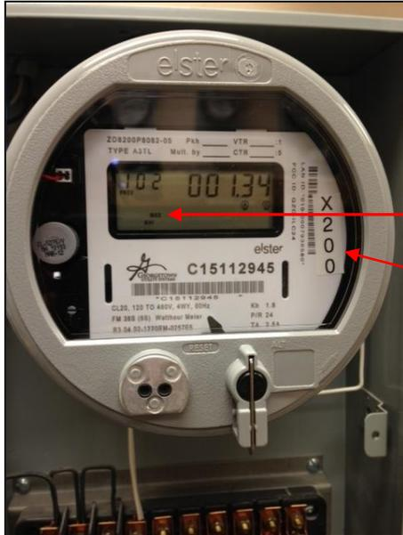
This screen is indicated by MAX KW in the lower left corner of the screen. The peak kW will always have a decimal, and is reset to 00.00 after each monthly reading is taken
